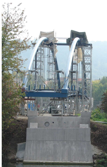
Endmontage am Ufer
